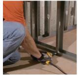
Screw studs to top and bottom runners using 7/16" pan screws.
