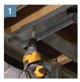
Attach ceiling runner to bottom of joist or truss.
