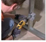
Snap in grommets for electric and plumbing.
