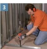
Attach floor runner using concrete anchors.
