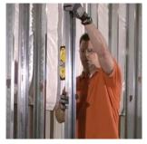
Twist studs into place. Make sure studs are level and knockouts/punch-outs are aligned.
