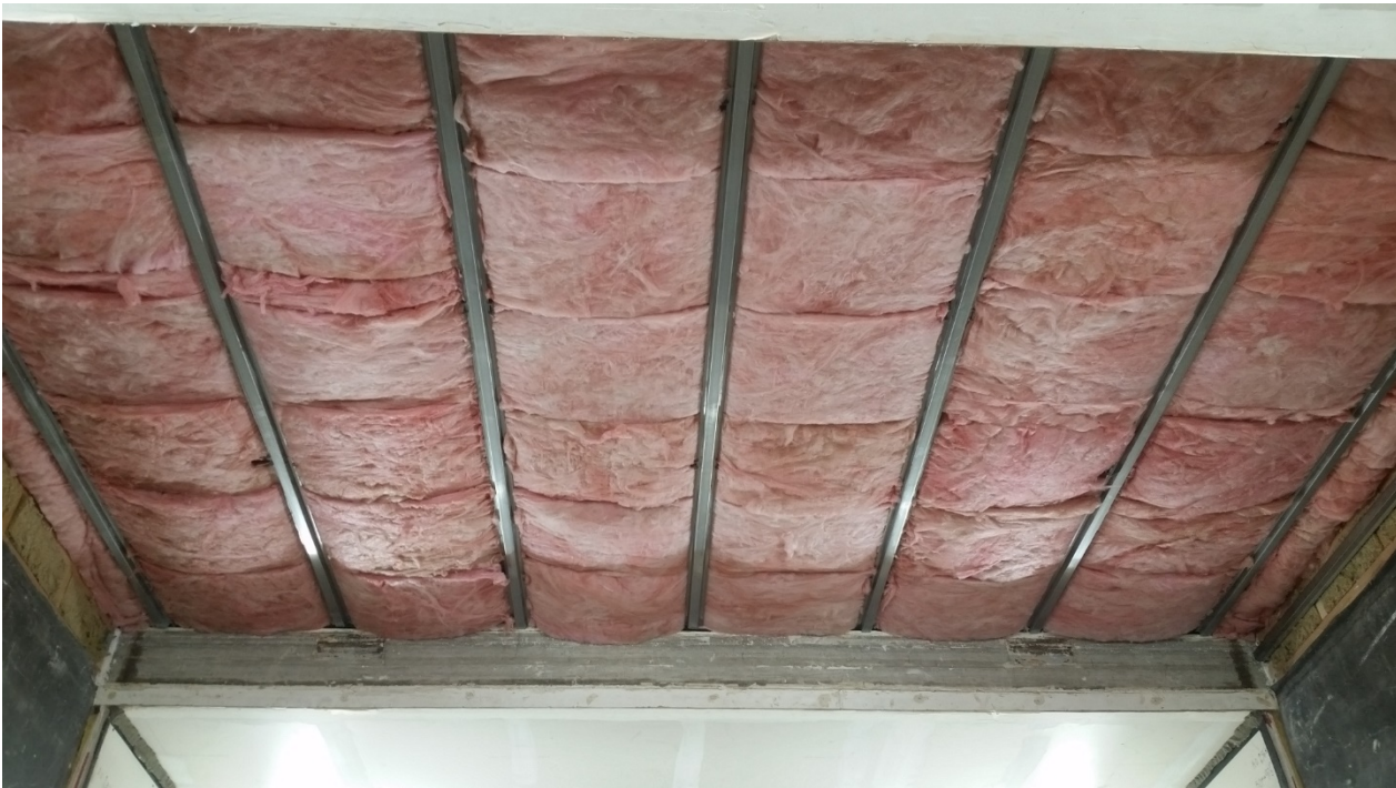
Figure 8 – Furring channel and insulation installed below slabs
