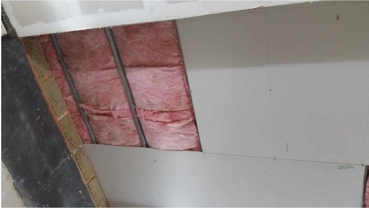
Figure 9 – First layer of gypsum board partially installed
