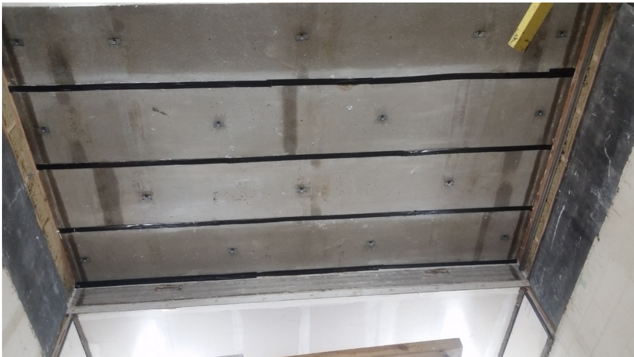
Figure 6 – Isolating clips installed to bottom of concrete slabs
