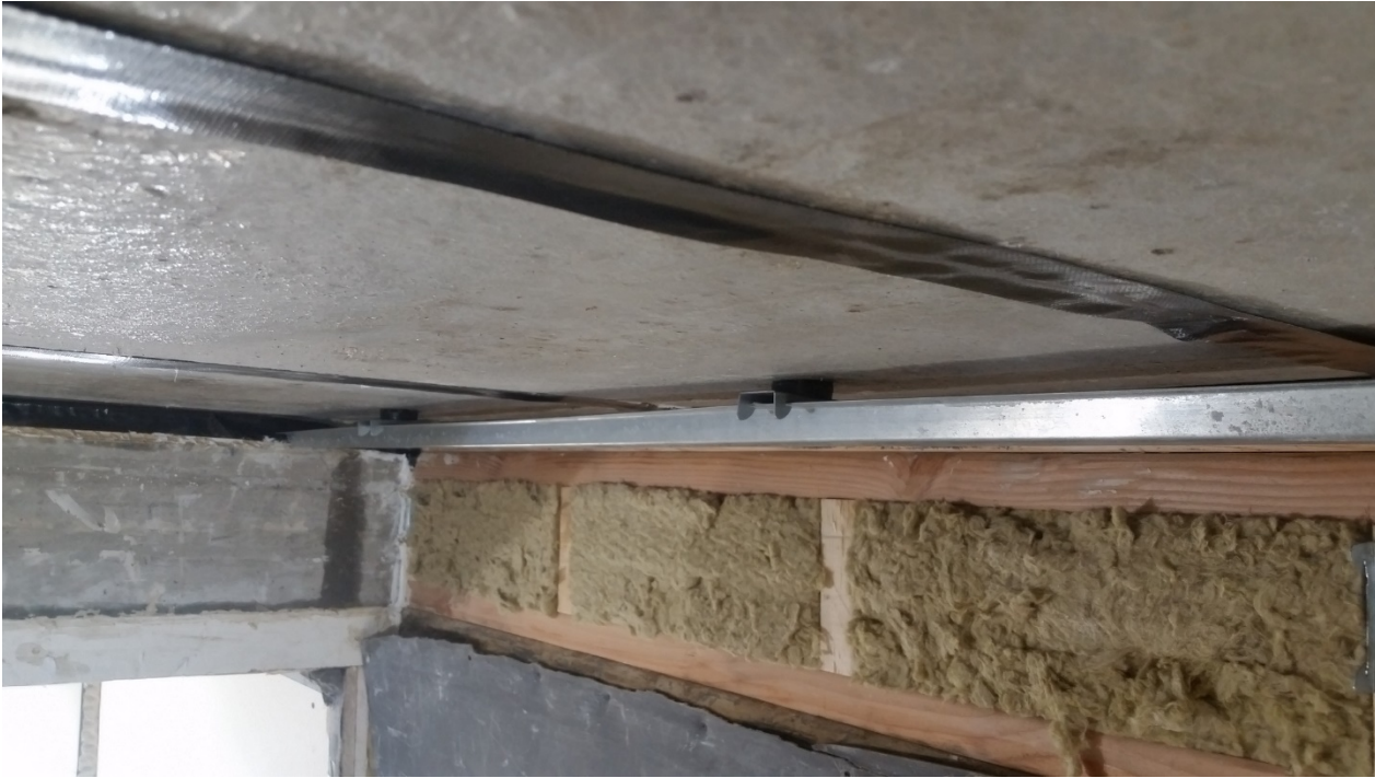
Figure 7 – Furring channel installed on isolating clips
